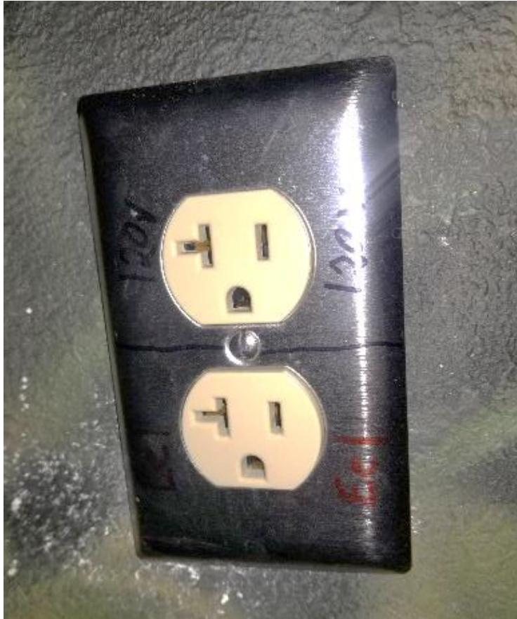
Figure 2. Divided outlet. 120V plug on top, Eel powered plug on the bottom.
