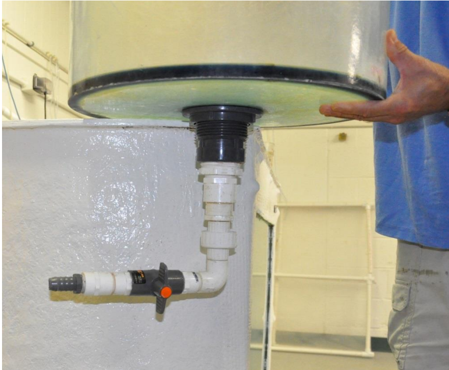
Figure 2: A close-up of the 90° drain valve plumbed into each grow-out tube.
