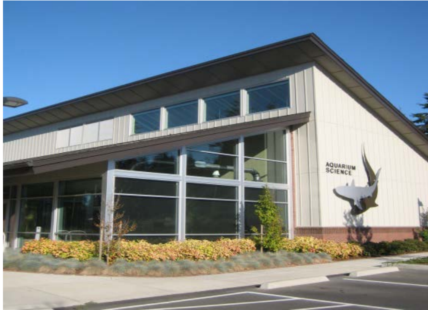
The 9,200 square foot Aquarium Science building was completed during the summer of 2011. The facility offers laboratory experiences to students in the program.
