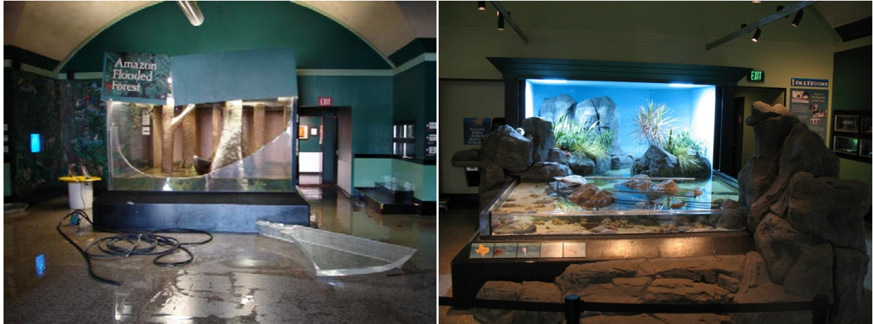
Figure 4: The aquarium’s invertebrate touch tank in 2007 (left) and 2010 (right). The tank was originally a 10,000 gallon Amazon exhibit that experienced a “technical fault in the operating device”, or as we say in south Dallas, “it blew the &@!# up”. The tank was remodeled into a touch pool making use of the existing concrete base and approximately 8” of the original acrylic. Photo (left) by Eric Julius.
