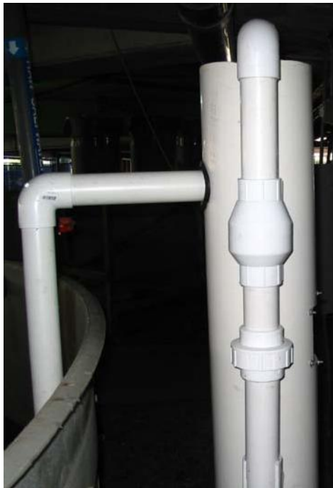
Figure 2. Side view of fluidized bed filter with influent and effluent lines shown.
