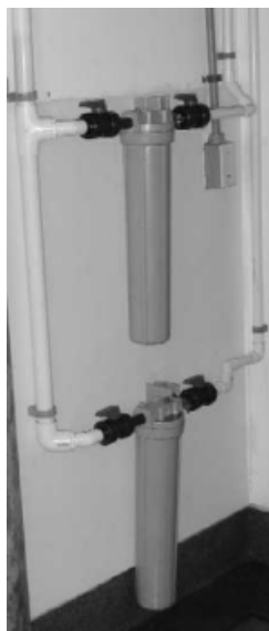
Figure 1: Picture of the topside portion of the autofeeder. The incoming line is the one on the left and feeds into the two 20" filter housings. The lines on the right travel to the exhibit.
